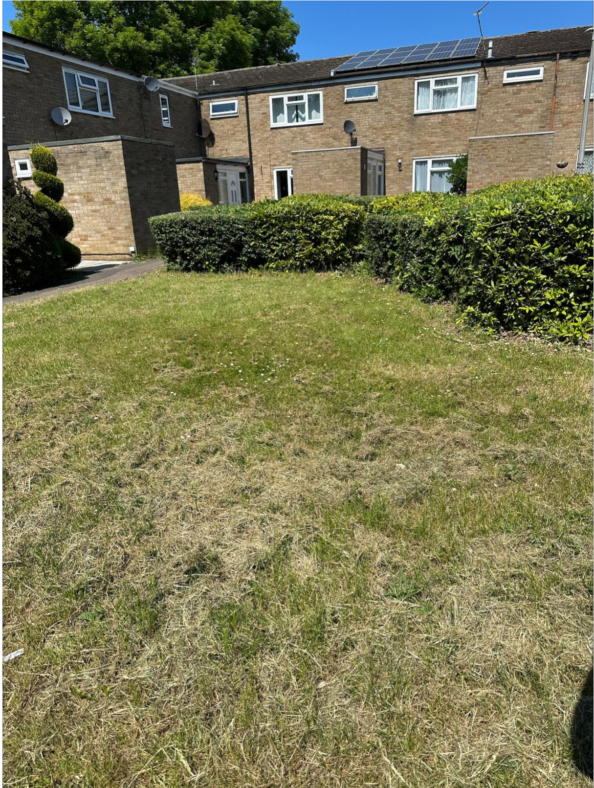
Coventry Close before works
