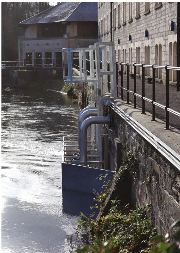
The water source heat pumps at Ebley Mill, Stroud
