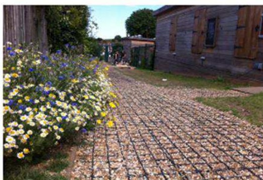
Rosendale Allotment before (Top) and after (Bottom) with new permeable surface.
